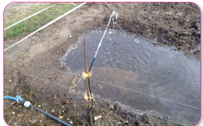
A wallow being replenished via an individual valve off of the main pipeline
