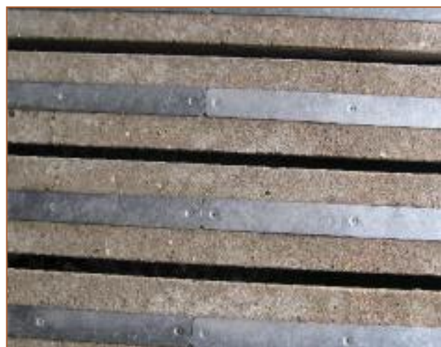
Slot closure insert after four months use
