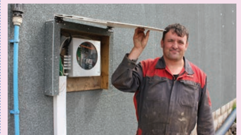
CO2 monitoring system in new finisher building on David Goodier's Focus Farm
